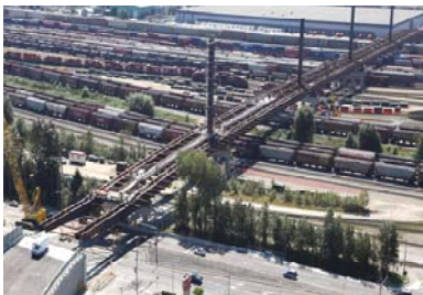
The launch of Coast Meridian Overpass nearing its final location
